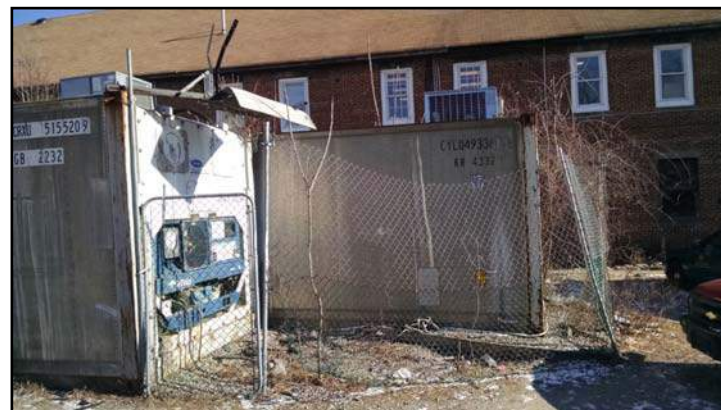
Abandoned refrigeration units with exposed wiring on litter-strewn lot with deteriorated fencing
