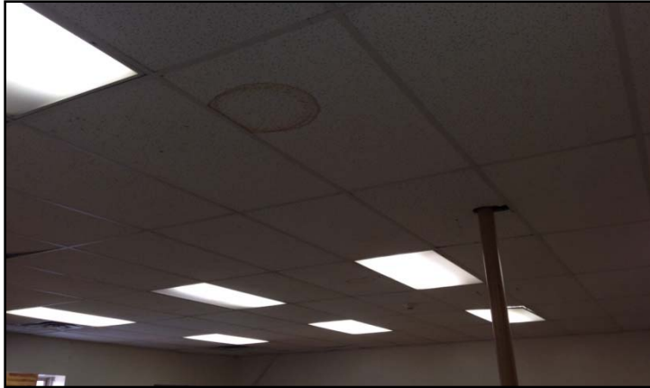
Evidence of water infiltration and compromised structural integrity of roof Note lack of fire suppression in school
