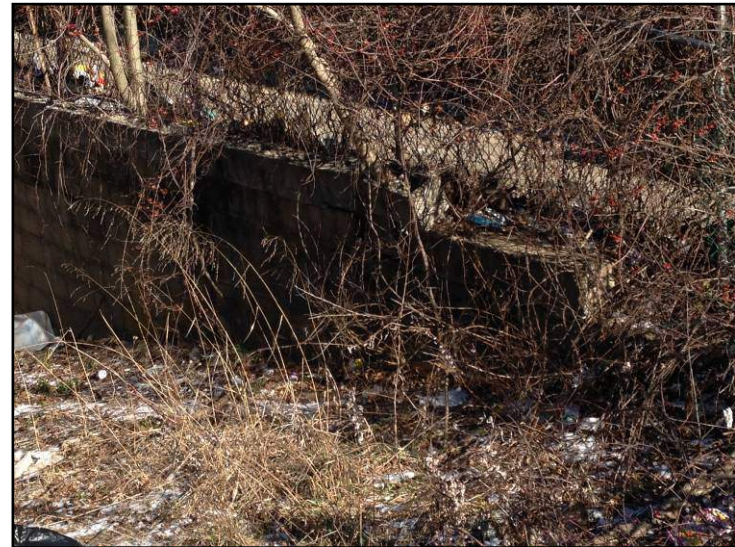
Bulging & deteriorated retaining wall at overgrown and litter-strewn loading dock
