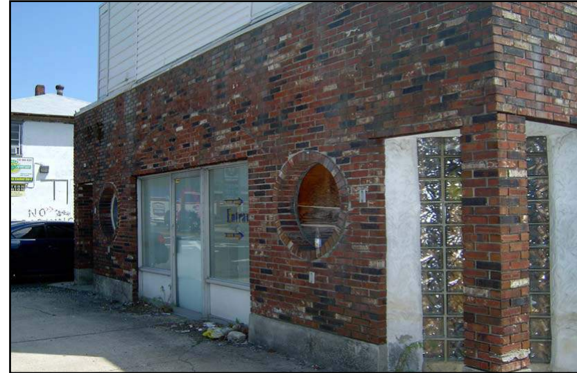
2007 Main Street View (Looking East) Building Since Demolished 162
