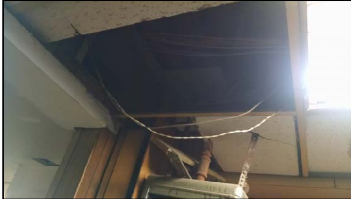
Exposed electrical wires
