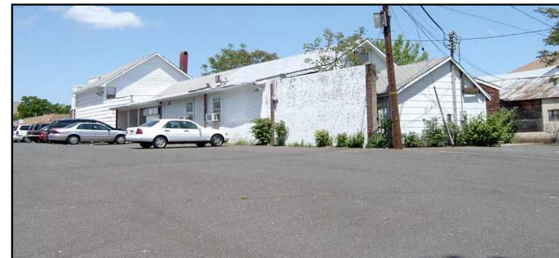
2007 Rear View (Looking Northeast) Building Since Demolished 162
