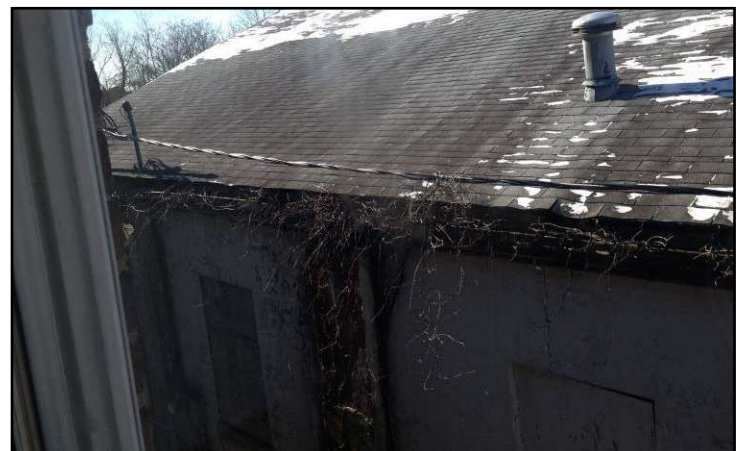
Buckled roof, clogged & damaged gutters and exposed & deteriorated structural member
