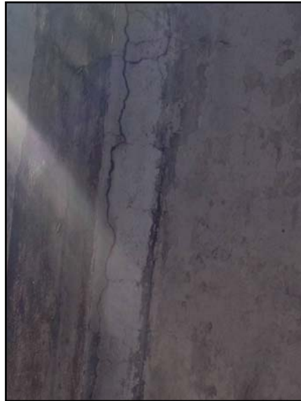
Cracked masonry siding
