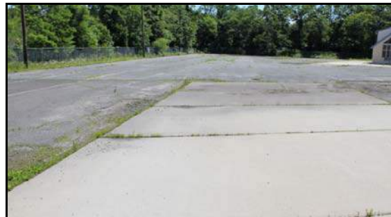
2014 Interior View (Looking East)
