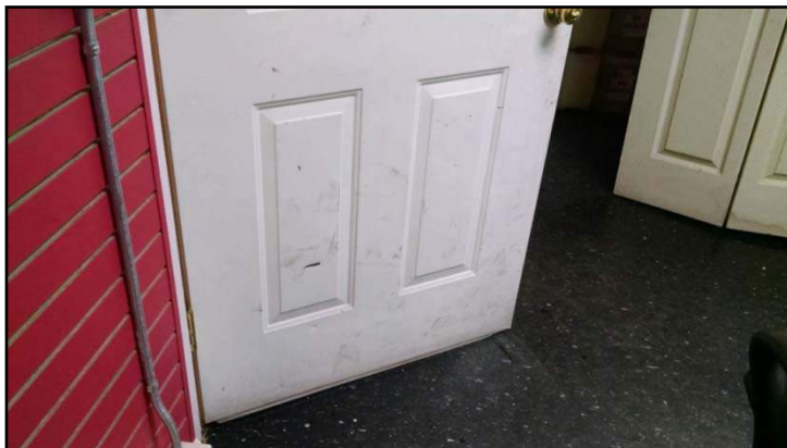
Nonfunctional 1 st floor doors (do not fully open) to secondary means of egress
