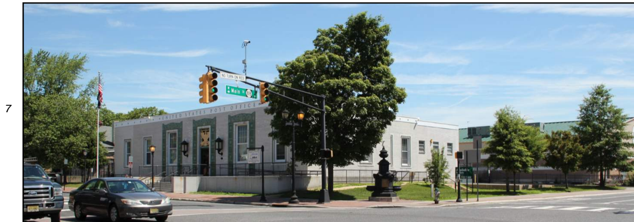
2014 Main Street View (Looking Northwest) from Intersection
