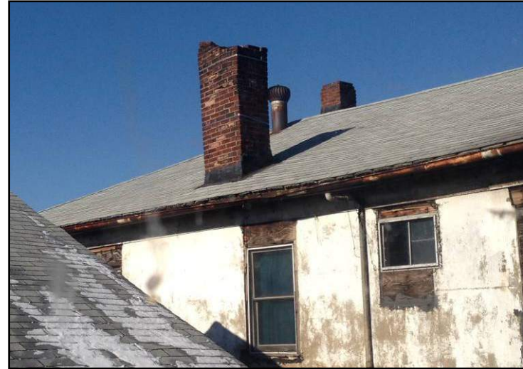
Damaged / deteriorated chimney, deteriorated soffits & masonry siding (exposing brickwork)
