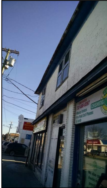
Missing / deteriorated soffits, broken down spouts & unsecured exterior wires
