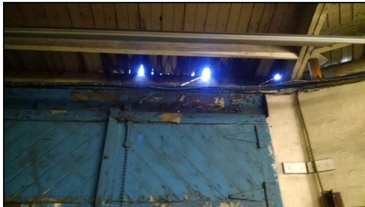
Deteriorated / damaged roofing
