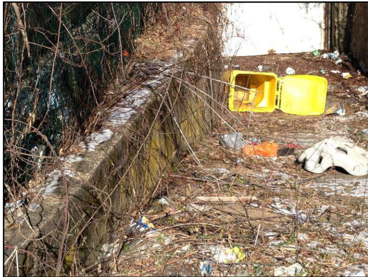
Bulging & deteriorated retaining wall at overgrown and litter-strewn loading dock
