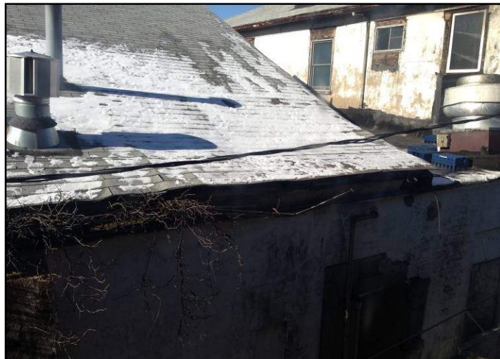
Buckled roof, deteriorated soffit, damaged & clogged gutters and deteriorated masonry siding (exposing brickwork)
