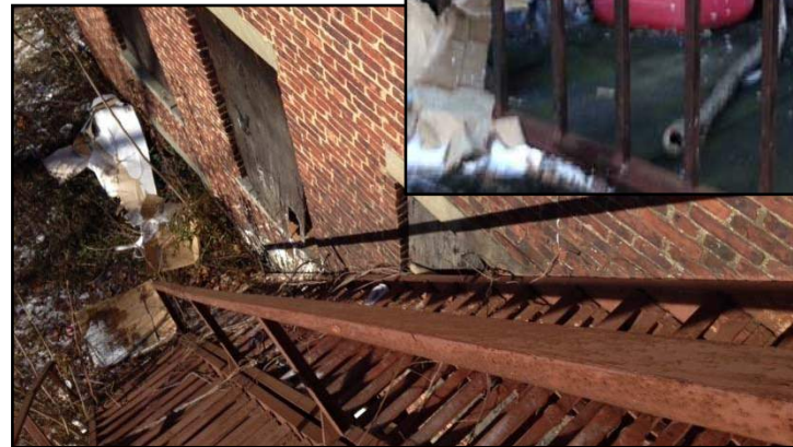
Litter, debris and abandoned gasoline container at base of (school) fire escape
