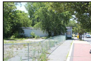
2014 Interior View Looking South
