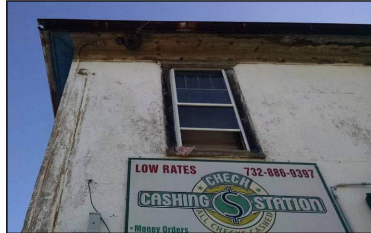
Missing / deteriorated soffits, broken down spouts & unsecured exterior wires
