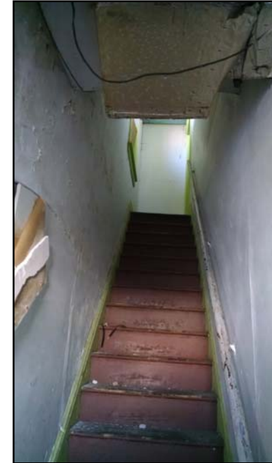
Dilapidated staircase, walls & ceiling and exposed wiring at secondary means of egress from 2 nd floor school
