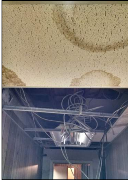
Evidence of Water infiltration in 1 st floor ceiling with exposed electrical wiring
