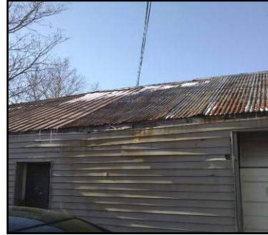
Buckled metal roof, damaged siding & damaged and clogged gutters on garage workshop with improperly fitted / installed garage door
