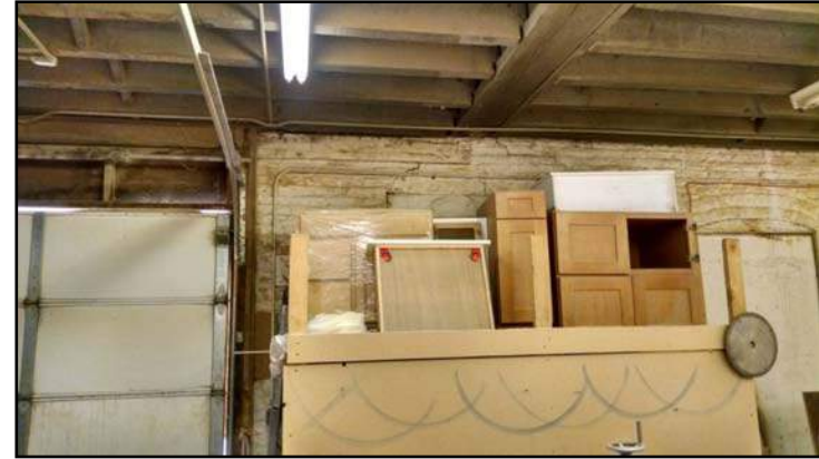
Numerous cracks & mold in/on 1 st floor structural (supporting) walls
