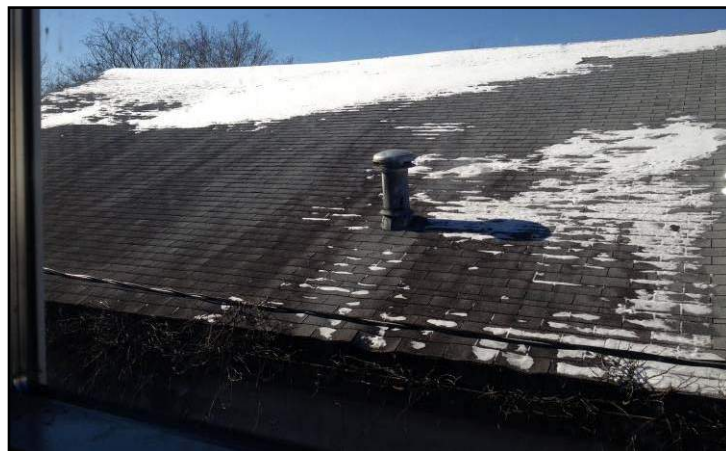
Buckled roof & deteriorated soffit
