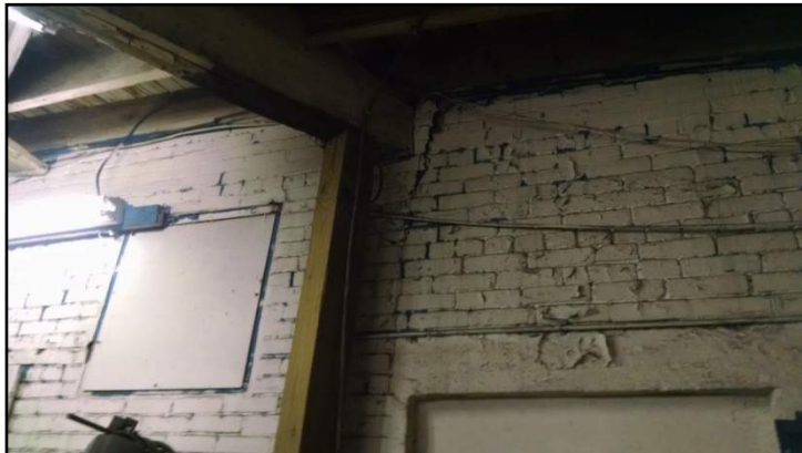
Numerous cracks in 1 st floor structural (supporting) walls
