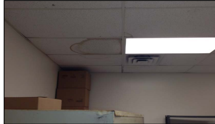
Evidence of water infiltration and compromised structural integrity of roof Note lack of fire suppression in school
