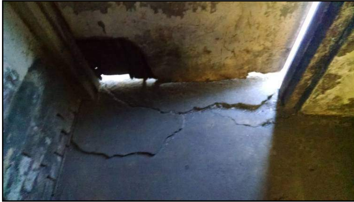
Deteriorated & unsecured exterior door
