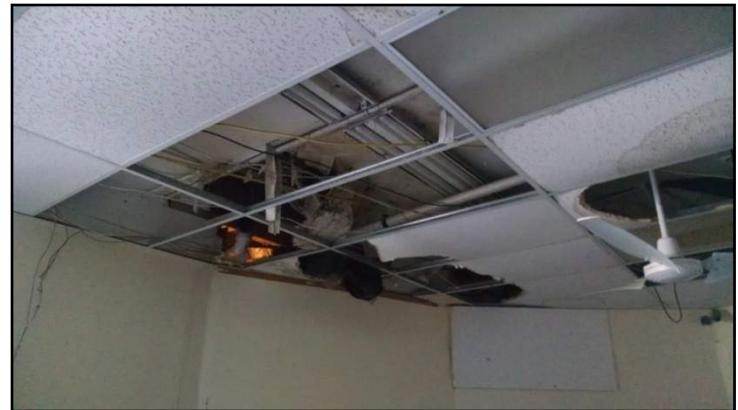
Exposed electrical wiring and abandoned light fixtures above 1 st floor drop ceiling
