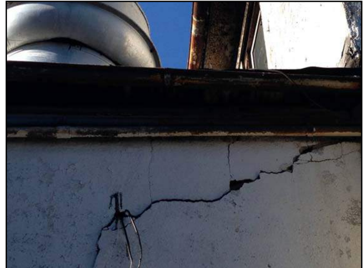
Cracked masonry siding & deteriorated soffit
