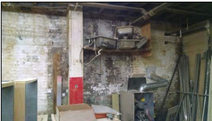
Numerous cracks & mold in/on 1 st floor structural (supporting) wall
