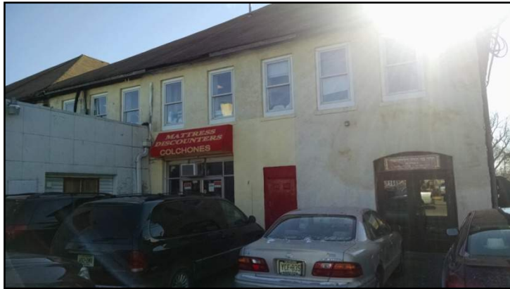
Missing soffits, broken gutters & blocked access to building
