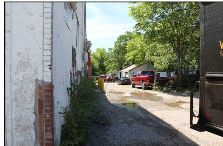
Standing water in uneven, potholed, gravel driveway / side yard
