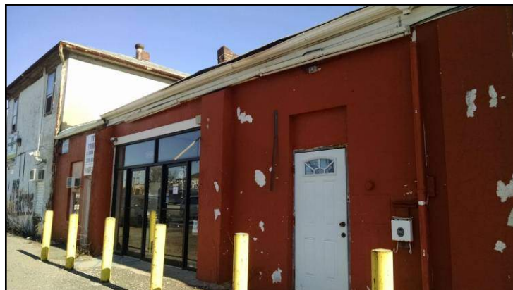
Exterior paint peeling (evidence of water damage, numerous cracks and broken downspouts)
