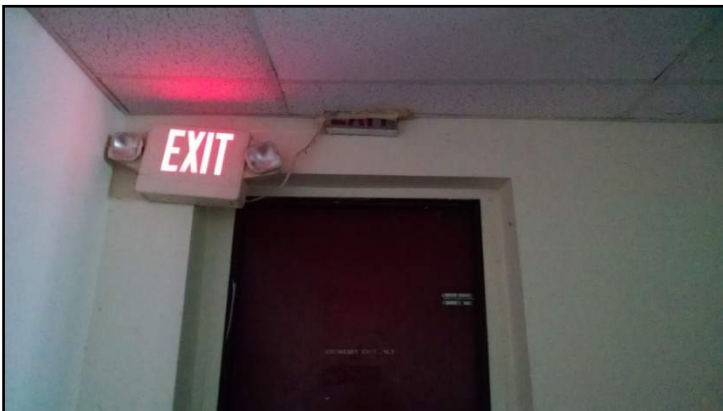
Exposed electrical wires feeding unsecured exit sign
