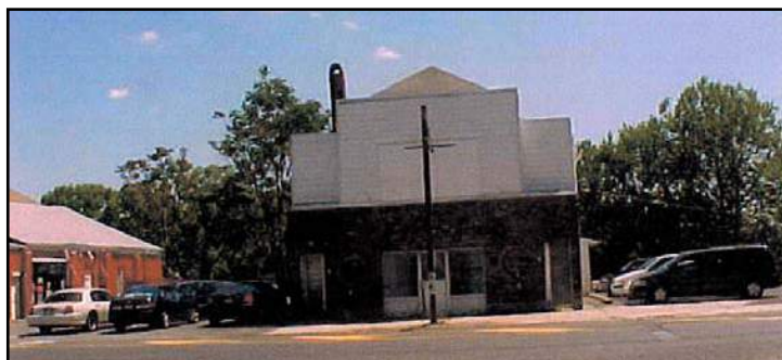
2007 Main Street View (Looking East) Building Since Demolished 162
