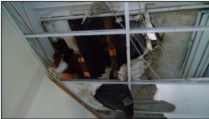
Exposed electrical wiring and abandoned light fixtures above 1 st floor drop ceiling
