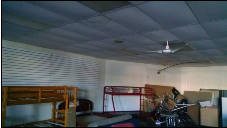
Evidence of water infiltration in 1 st floor ceiling (note exposed electrical wiring ~ top left) (note lack of Fire Suppression throughout)
