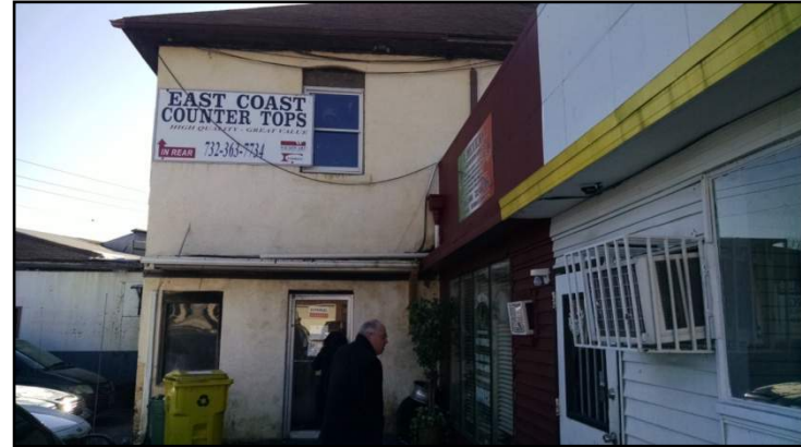
Missing soffits, broken gutters & unsecured wires
