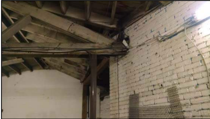
Deteriorated (broken & rotted) roof / ceiling trusses, supported by make-shift wood / steel columns (note hole in roof ~ top right)
