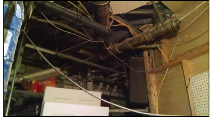
Exposed electrical wiring and plumbing (1 st floor)
