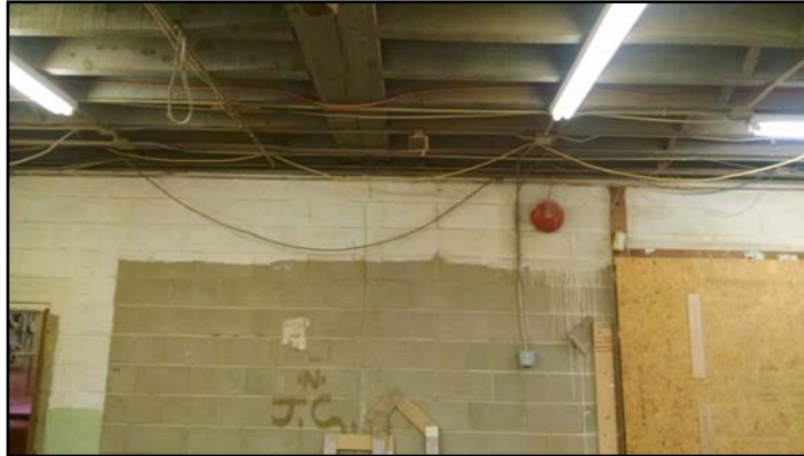
Large crack under main beam supporting 2 nd floor school
