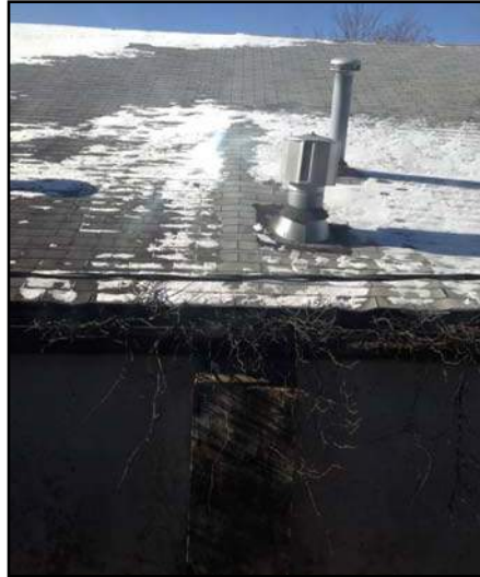
Buckled roof, deteriorated soffit, damaged & clogged gutters & exposed and deteriorated structural member
