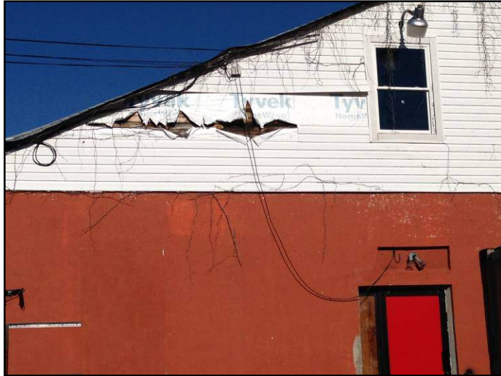
Damaged siding, unsecured wires & deteriorated roofline
