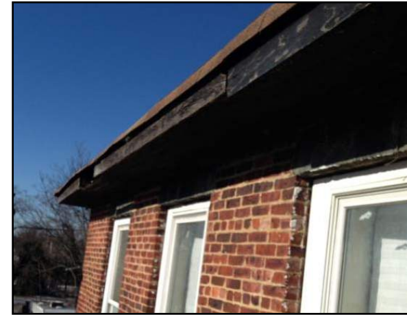
Deteriorated soffits at roof eaves
