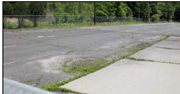
2014 Interior View (Looking Northeast)
