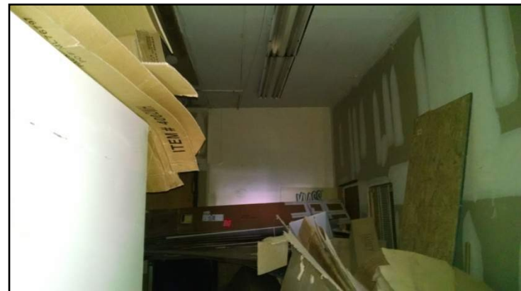
Debris strewn throughout building
