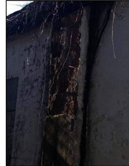
Exposed & deteriorated structural member
