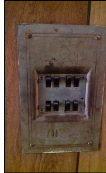
Obsolescent Electrical panel with evidence of scorching
