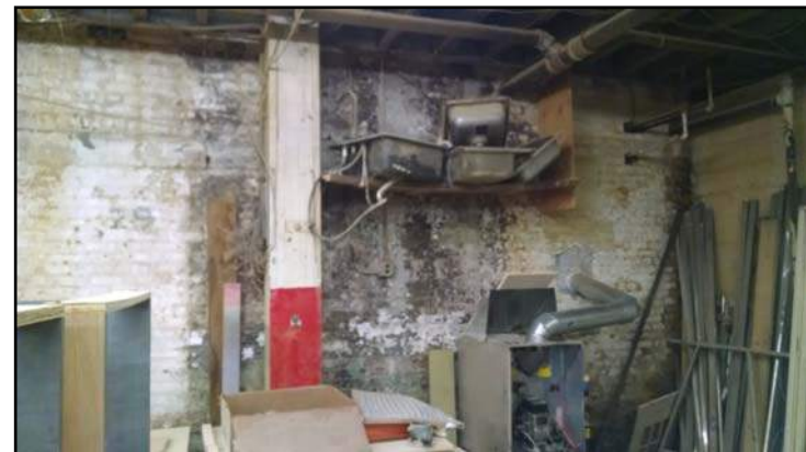
Numerous cracks & mold in/on 1 st floor structural (supporting) wall
